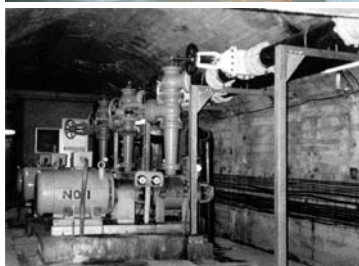
Kanmon Undersea Tunnel drainage equipment SL-NBP-200
