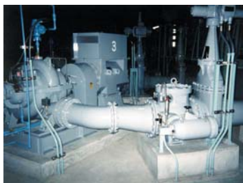
Filtration plant Dashpot Type Check Valve SL-SN-400B
